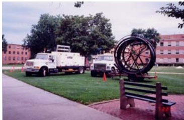
Main campus commons irrigation system under construction
