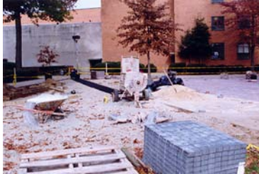
Existing student plaza under construction
