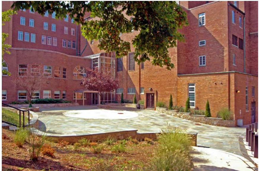
Design of Landscaped Student Plaza at New Addition of West Campus Law School
