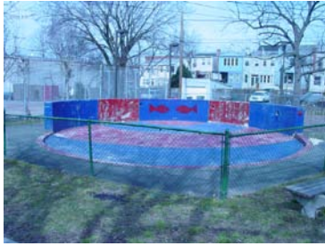
Existing Spray Park in Considerable Disrepair
