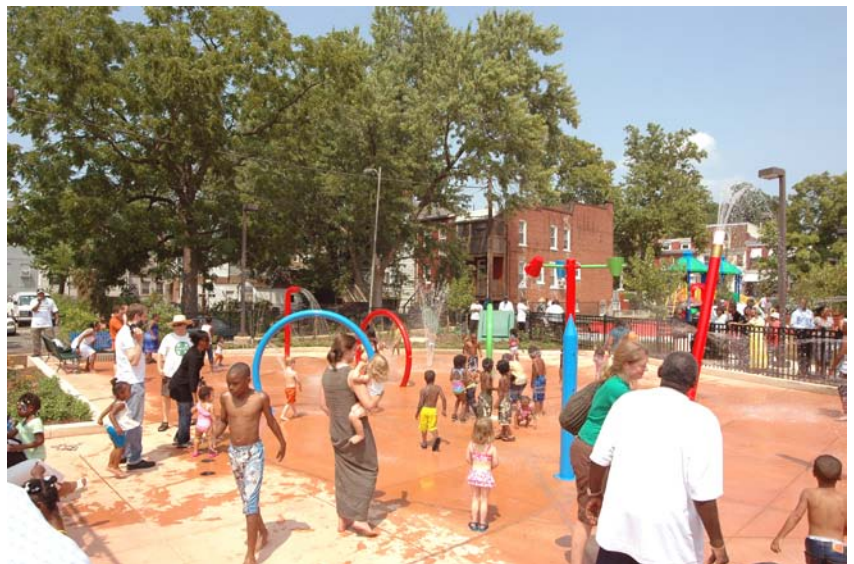
Installation of Spray Park with Interactive and Automated Features.
