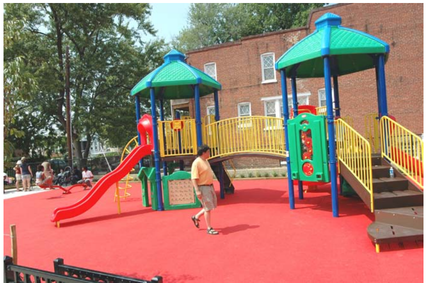
Installation of Playground Apparatus for ages 2-5
