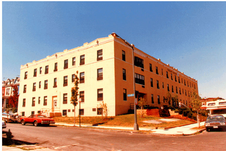
Fully Renovated Exterior and Interior of Two (2) Apartment Buildings into One (1) SRO Facility.
