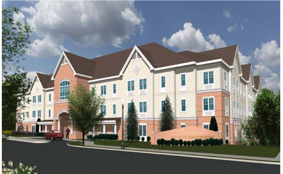
Eastgate Senior Residence Located on a Separate Site Landscaped with a Therapeutic Garden and Pedestrian Amenities for Outdoor Recreation
